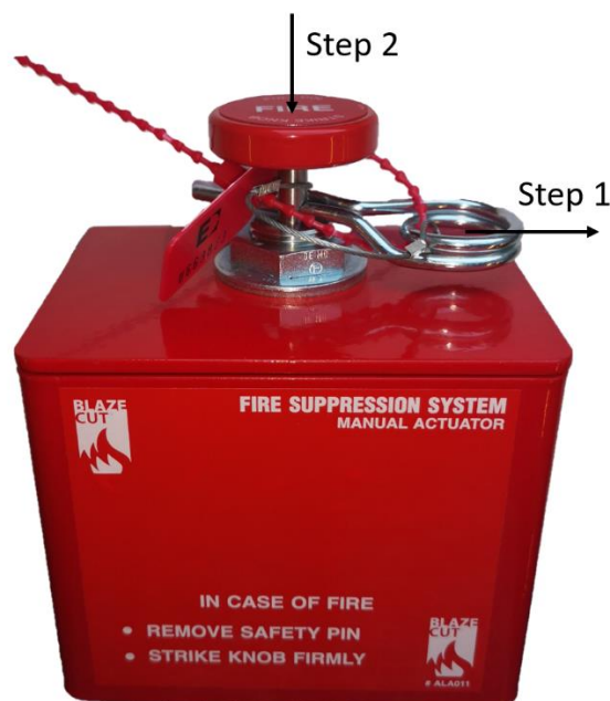
Procedure of manual activation
